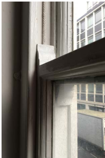
Modern single-glazed timber-framed sash (no glazing bars) Condition: Moderate. In need of redecoration and some repairs.
