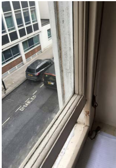
Modern single-glazed timber-framed sash (no glazing bars) Condition: Moderate. In need of redecoration and some repairs.
