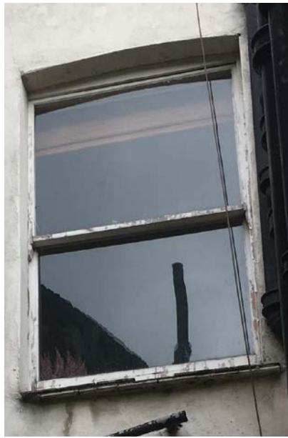
Modern single-glazed timber-framed sash (no glazing bars) Condition: Poor. In need of redecoration and extensive repairs.
