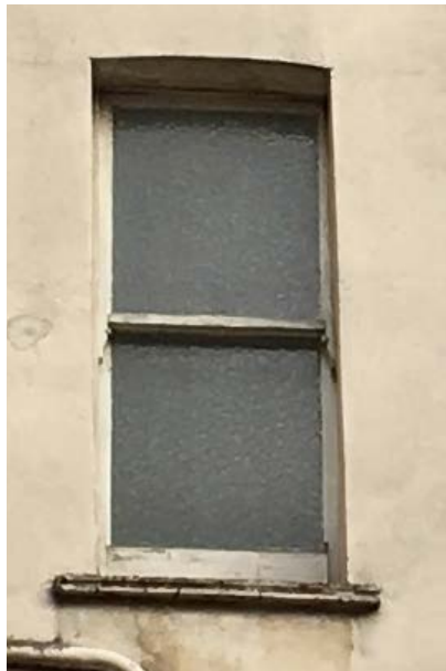
Modern single-glazed timber-framed sash (no glazing bars) Condition: Poor. In need of redecoration and extensive repairs.
