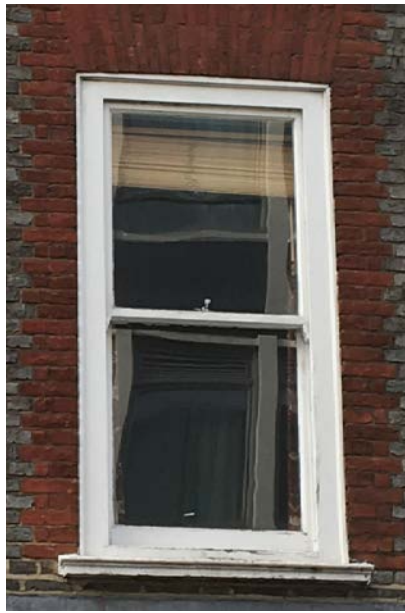
Modern single-glazed timber-framed sash (no glazing bars) Condition: Moderate. In need of redecoration and some repairs.
