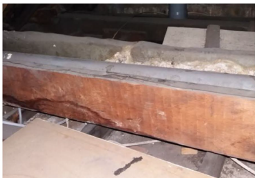
Modern machine-sawn collar with remnants of older timber behind
