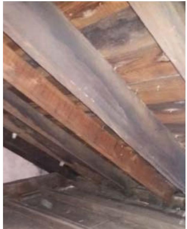
Variable sized rafters of different ages - all thought to not be original
