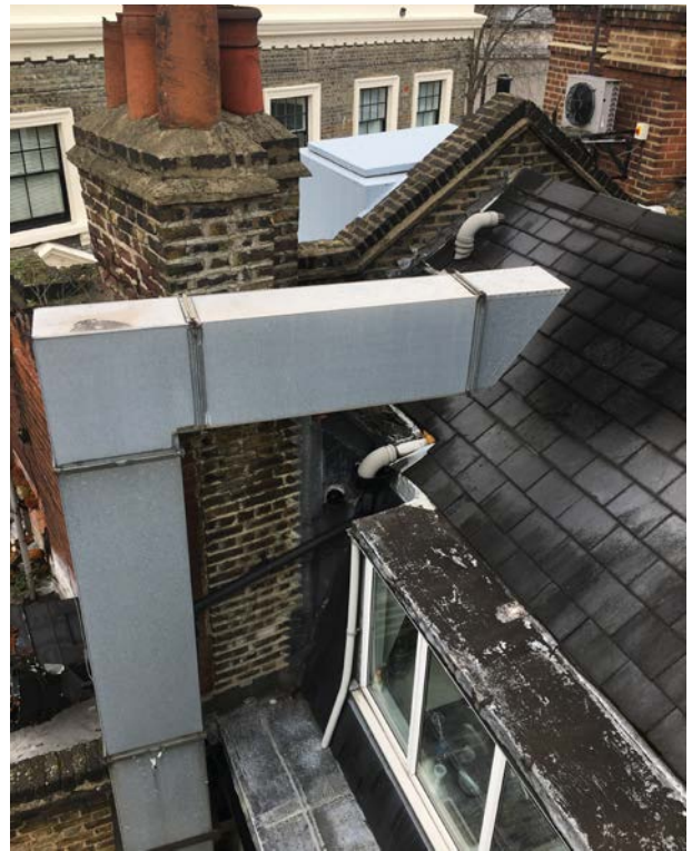
Vent extract from ground floor restaurant terminates towards rear roof slope
