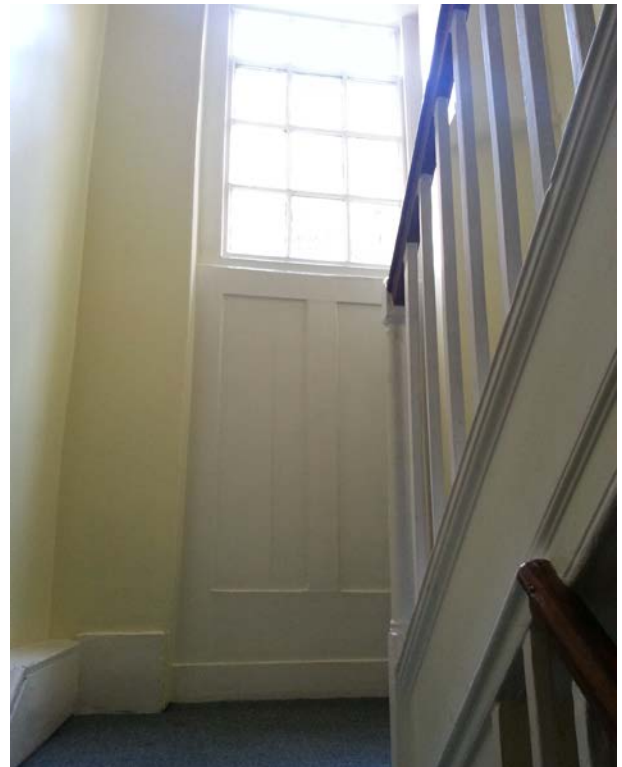
Stair at no. 46: short run of historic painted timber stringers, newels and balustrades
