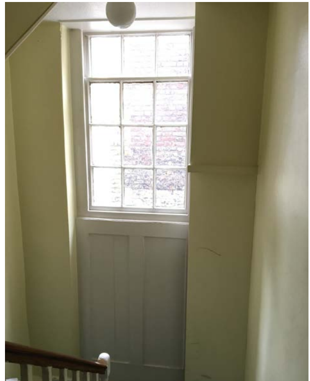
Services boxing-out partially obscuring historic window
