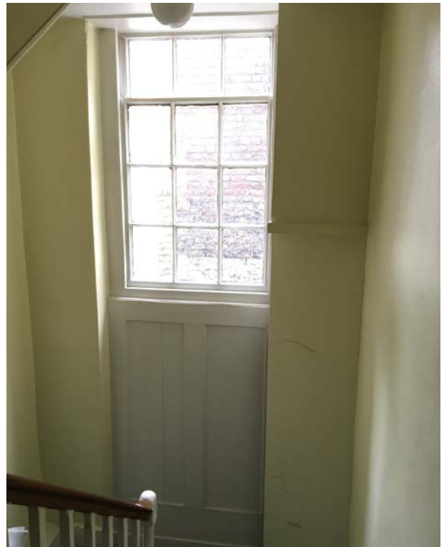
Internally, this has been truncated. Original timber panelling remains below.
