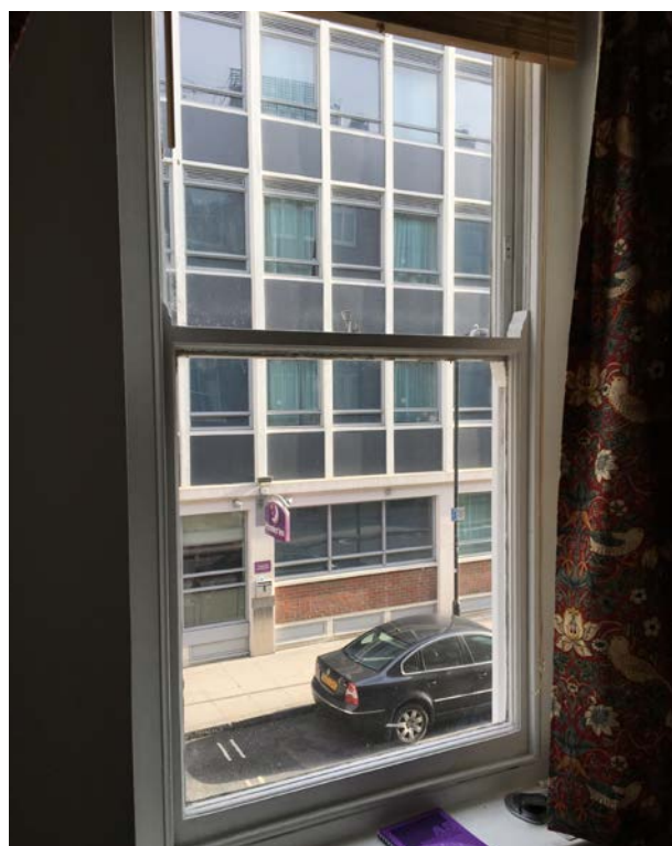
Recent timber sash windows to front facade at no. 46
