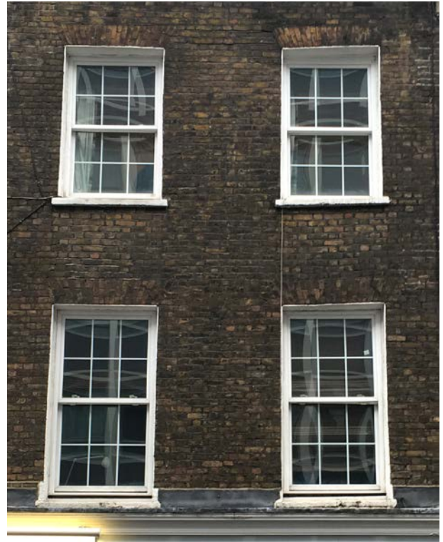
No 45: gauged yellow stock brick flat arches to recessed sashes
