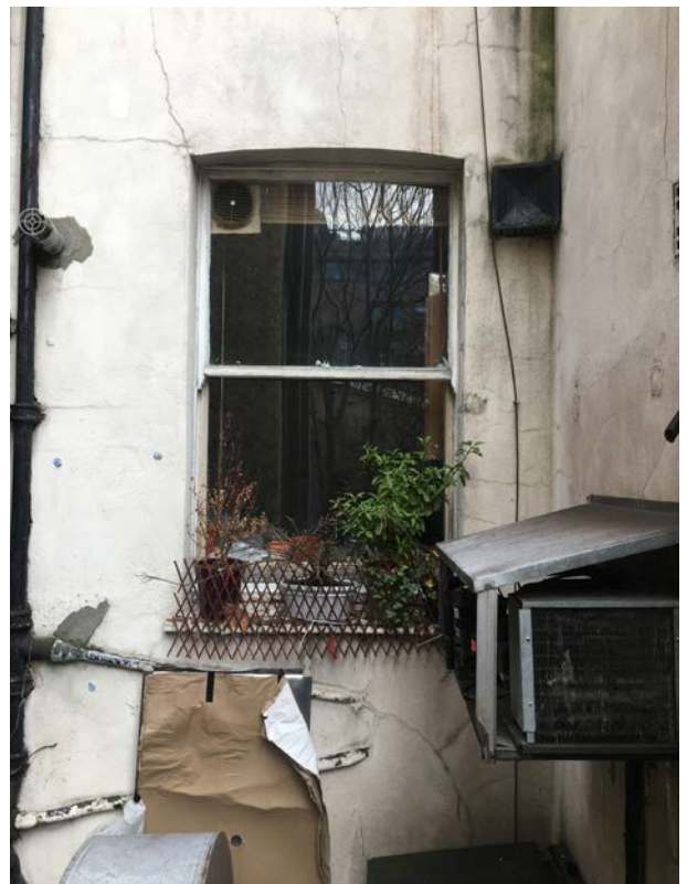
Recent timber sash windows to rear facade at no. 46
