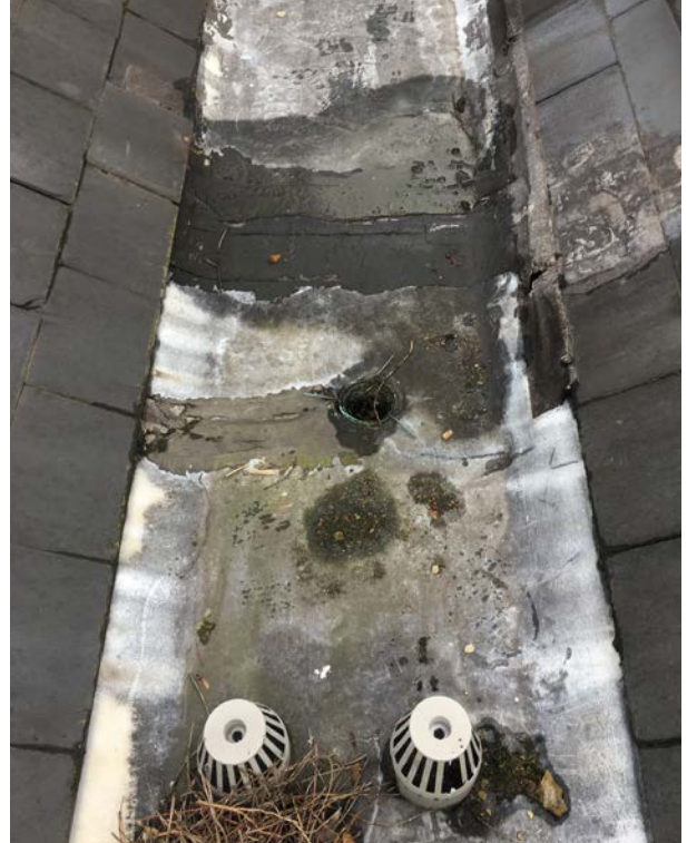
Poor quality lead valley which suffers often from flooding
