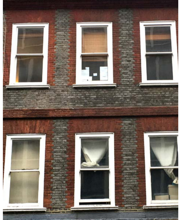
No 46: gauged red brick flat arches and red brick banding
