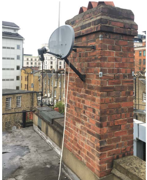
Repairs required to roof and party wall coping and redundant services to be removed
