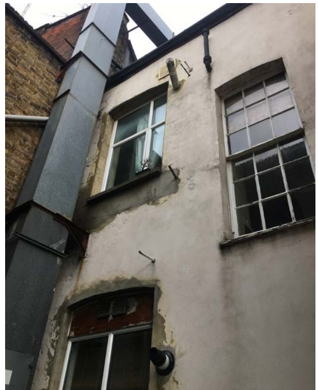
Unpainted and poorly executed render around windows and service penetrations
