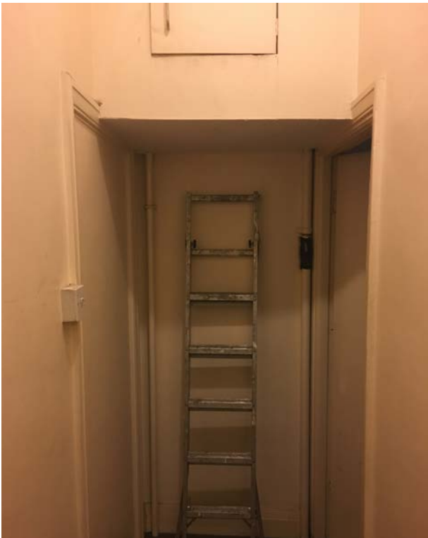
Bulkheads and service joinery interrupt door frames
