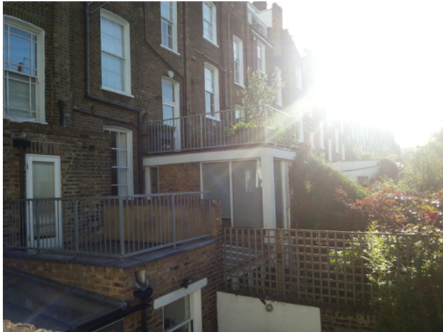
Rear of nos. 215 and 217 Gloucester Avenue view from Fitzroy Road
