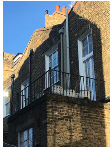
Rear of no. 131 Gloucester Avenue view from Fitzroy Road
