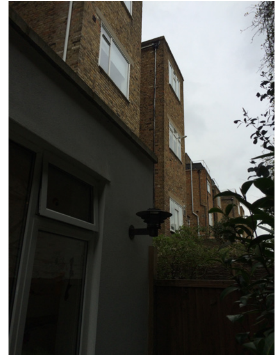
View from garden along rear elevation [looking North West]
