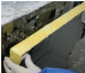
Isover CLIMCOVER slab installation
