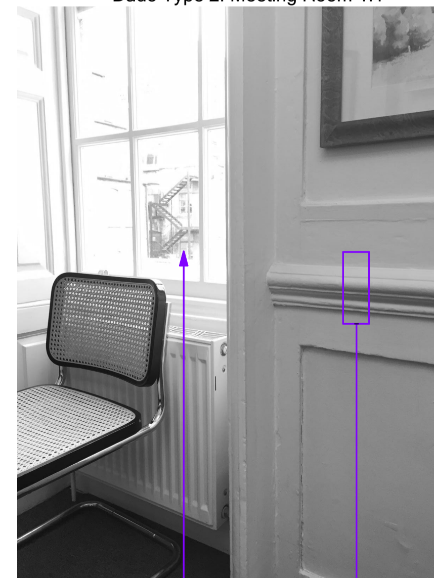
Window adjacent to meeting room jib door
