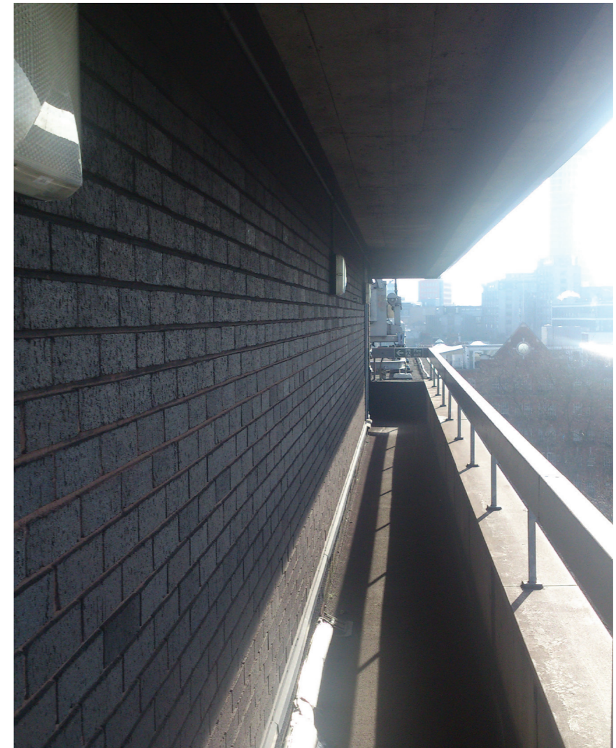
2- Existing wall where proposed new windows will be located
