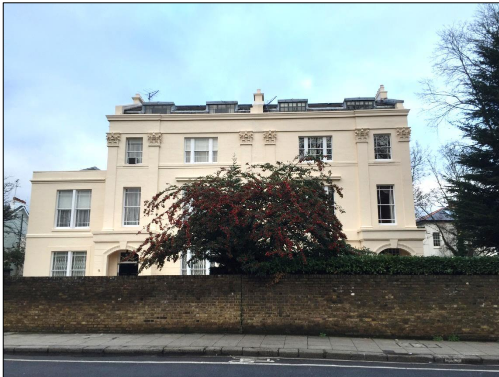
Photograph 2.2 (above): Nos. 8 and 9 Prince Albert Road, Front Façades. No. 9 (left) rebuilt in facsimile in late 1980s with two storey side 'extension'.
