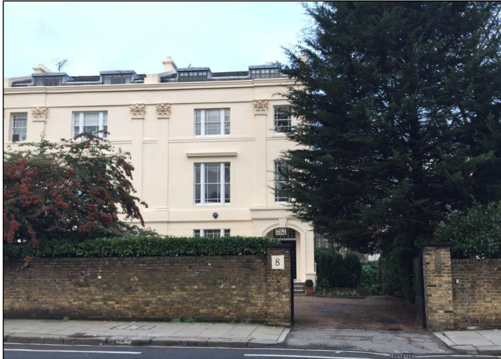
Photograph 2.1 (above): No. 8 Prince Albert Road, Front Façade.
