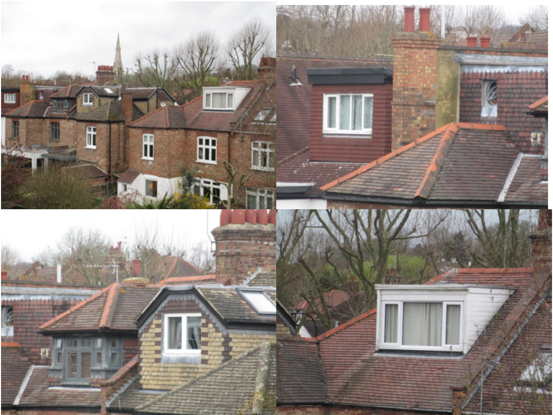
Rear dormers on south side of Swains Lane viewed from adjoining property in St Alban's Road
