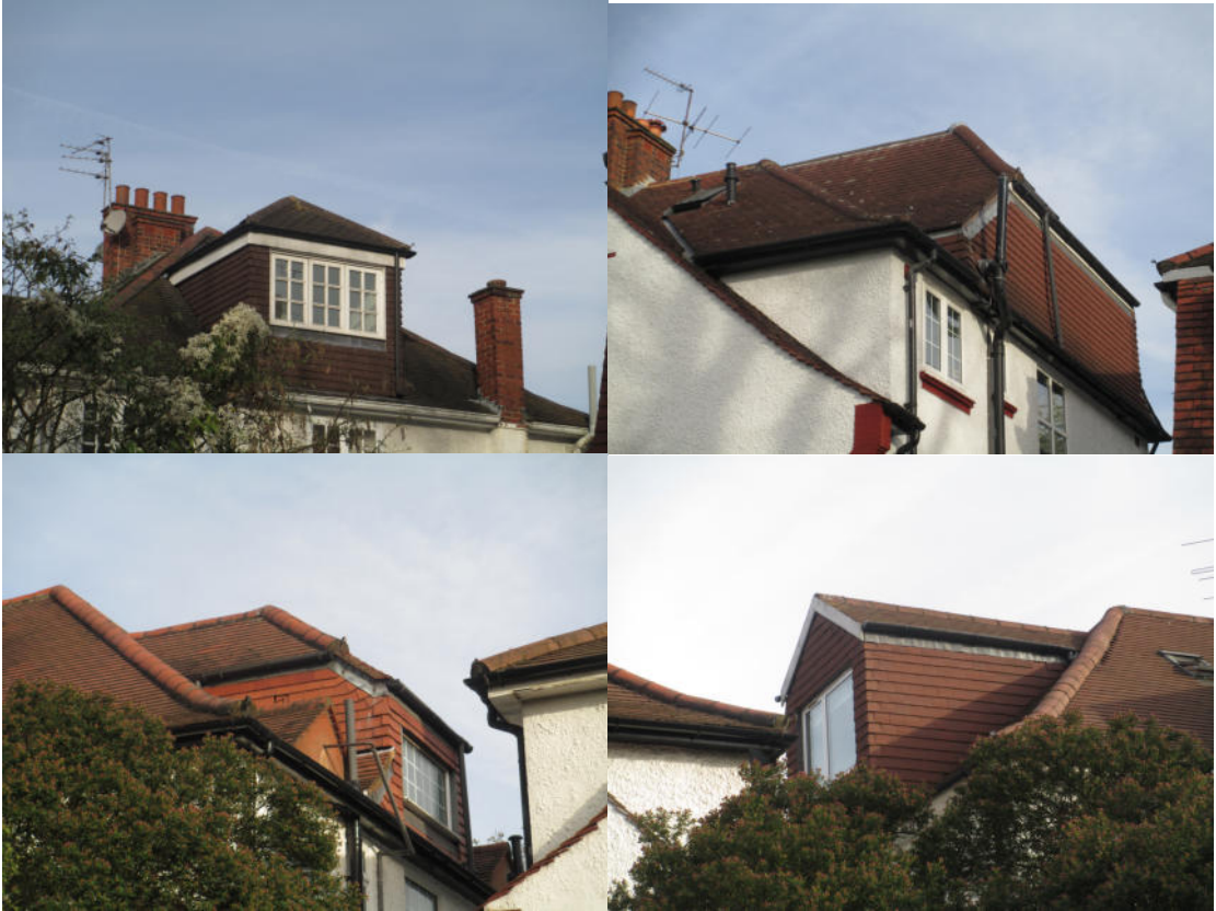
Side dormers on north side of Swains Lane viewed from the street
