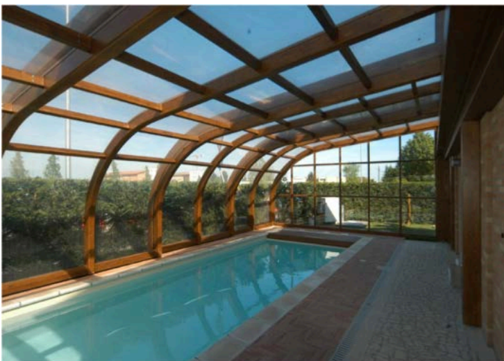
Example Glulam and polycarbonate pool enclosure
