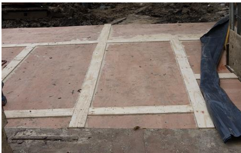
Figure 9. Plywood sheeting used as ground protection.
