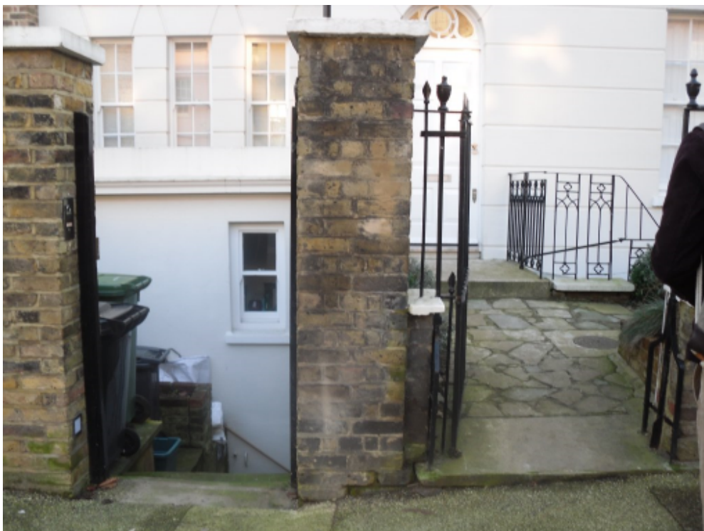
4. View of access to main house & side lightwell to be enclosed
