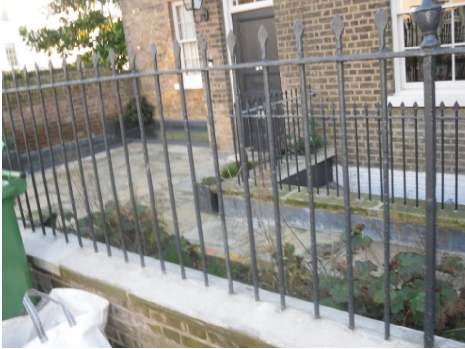
7. Similar enclosed front lightwell at no.34 Downshire Hill
