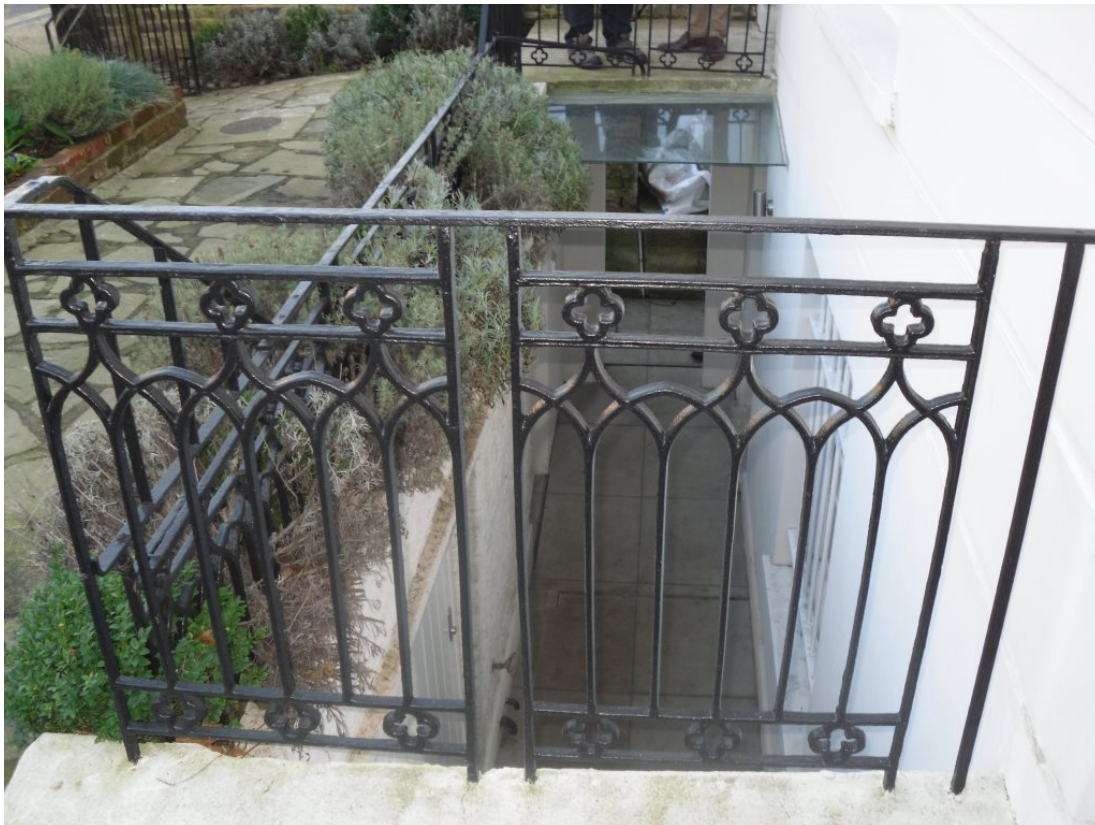
2. View of existing main Lightwell
