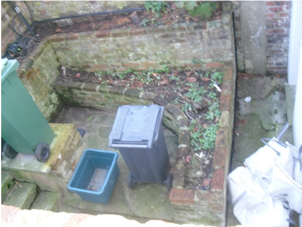
3. View of lightwell on north eastern side
