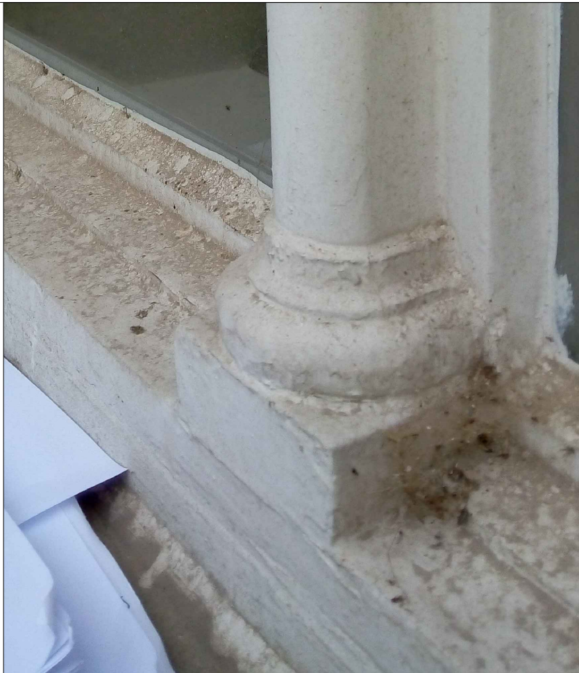
NORTH CLOISTERS EXISTING WINDOW Surveyed on 19/05/2016 by Andrei CIOREI & Jas NANDRA
