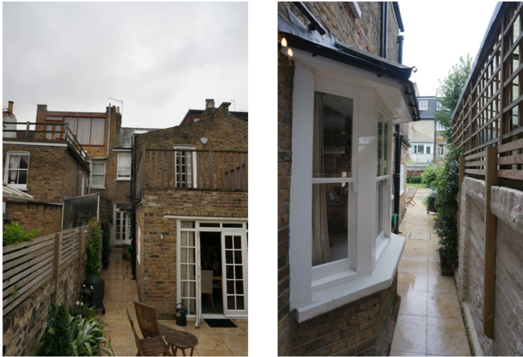
Views of existing side passway and back extension at 66 Solent Rd, dormer extension at neighbouring property 64 Solent Rd
