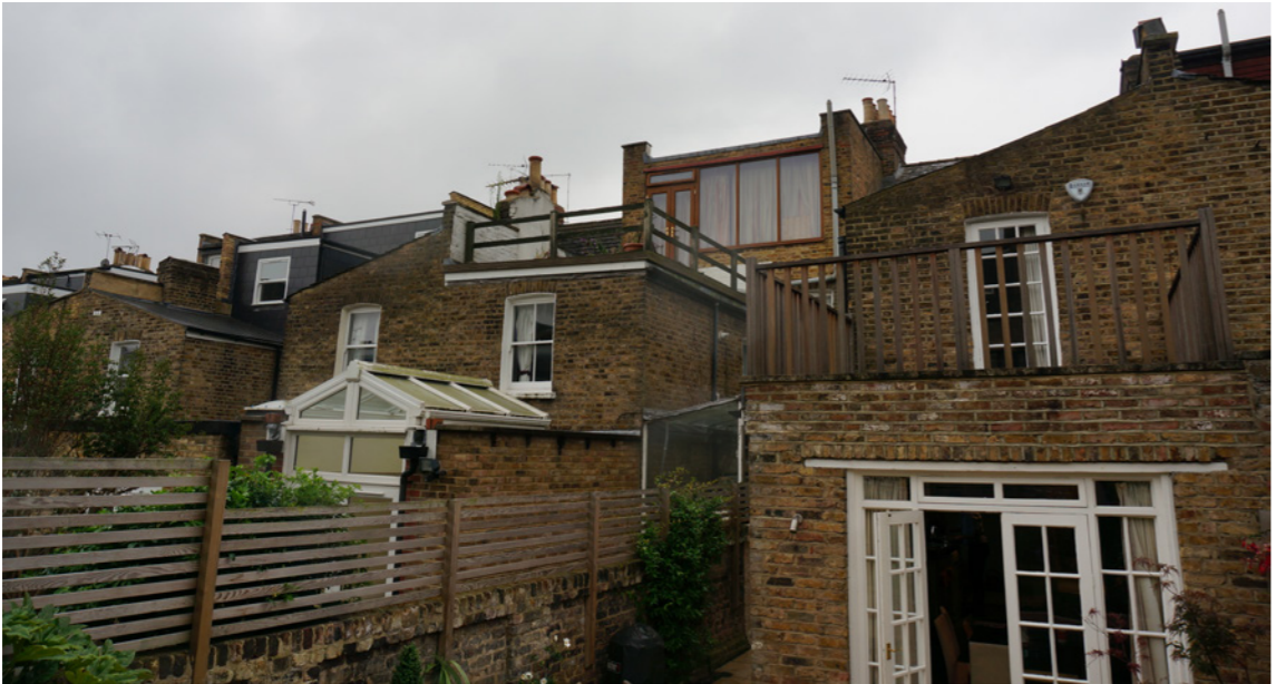
Photo 3 – Rear Elevation of No.64 (to left hand side of photo)
