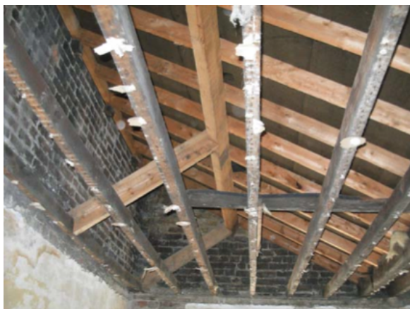
Fig.1 photograph of unapproved renovation works undertaken in 2013 showing the renewed roof timbers and clearly showing that the ceiling had been removed without consent by the previous owner.
