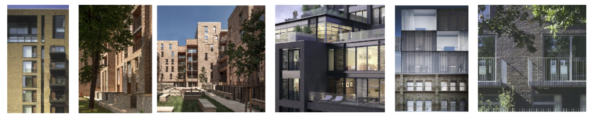
Windows and balconies with integral screening Architect: Allies & Morrison Varying reveals to articulate forms and massing Architect: Ponter Hudspith Upper storey flats glazed to the north and south with private terraces Lightweight, complementary upper storeys. Architect: Duggan Morris Projecting balconies - Flat steel section balustrades Architect: Tony Fretton
