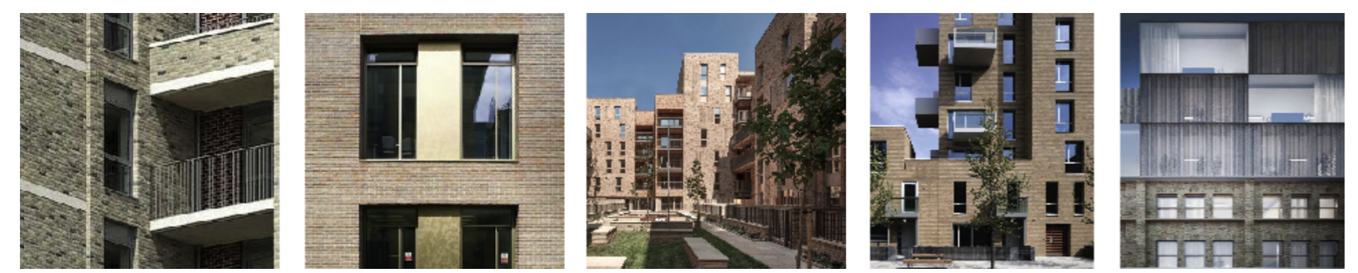
Mixed stock facing brick - contrasting tones Architect: PRP Architects Deep brick reveals with aluminium windows & panels Architect: Hawkins|Brown Varying reveals to articulate forms and massing Architect: Panter Hudspeth Stepping & recessed massing Architect: Allies and Morrison Lightweight, complementary upper storeys Architect: Duggan Morris
