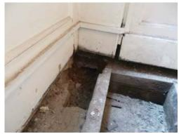
Rotten (missing) structural wall plate and beam end to first floor rear room
