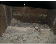
Photo 4: View of joists built into party wall.
