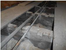
Photo 3: Notches to third floor rear room joists.
