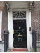
Existing front door showing existing door furniture. Water damage shown at base of timber pilasters
