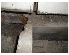
Photo 2: Rot to first floor beam end (beam A)
