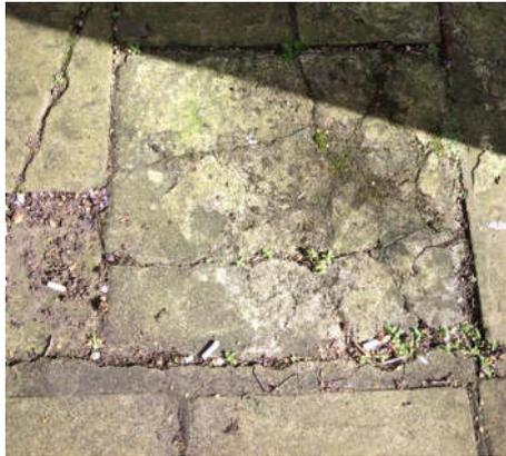
(4) Careful removal of concrete from surface of paviour, assessment of surface condition
