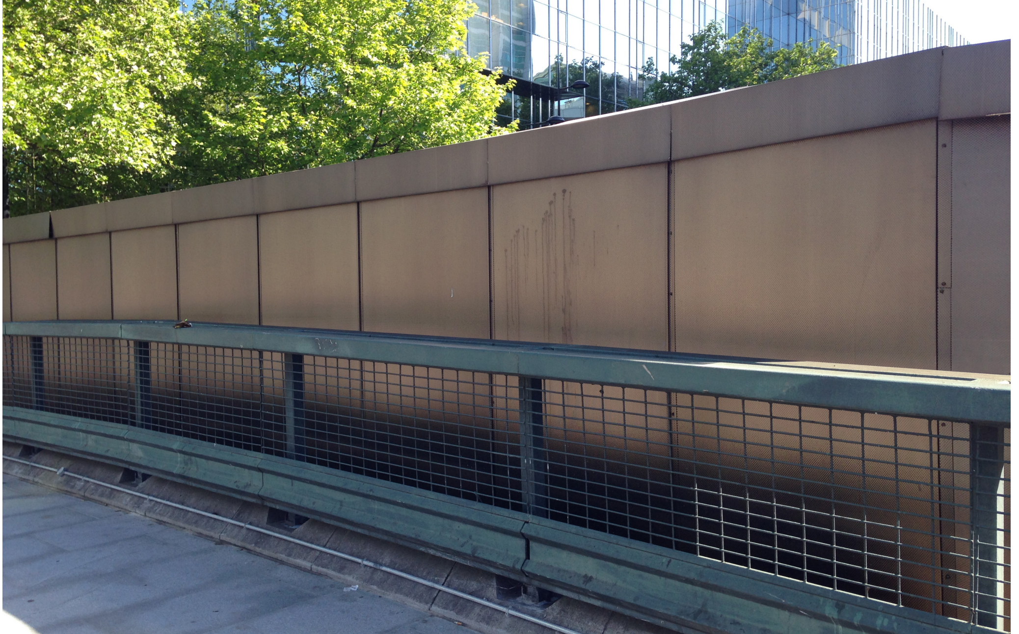
Euston Underpass Advertisements Rear Cladding Material
