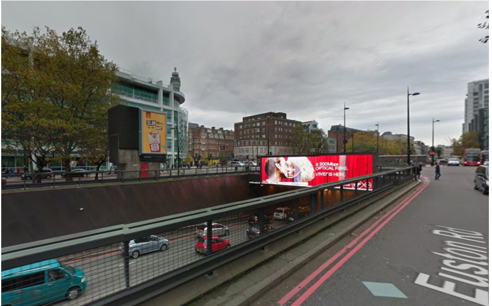
Euston Underpass Advertisement (Eastern Entrance) and P250
