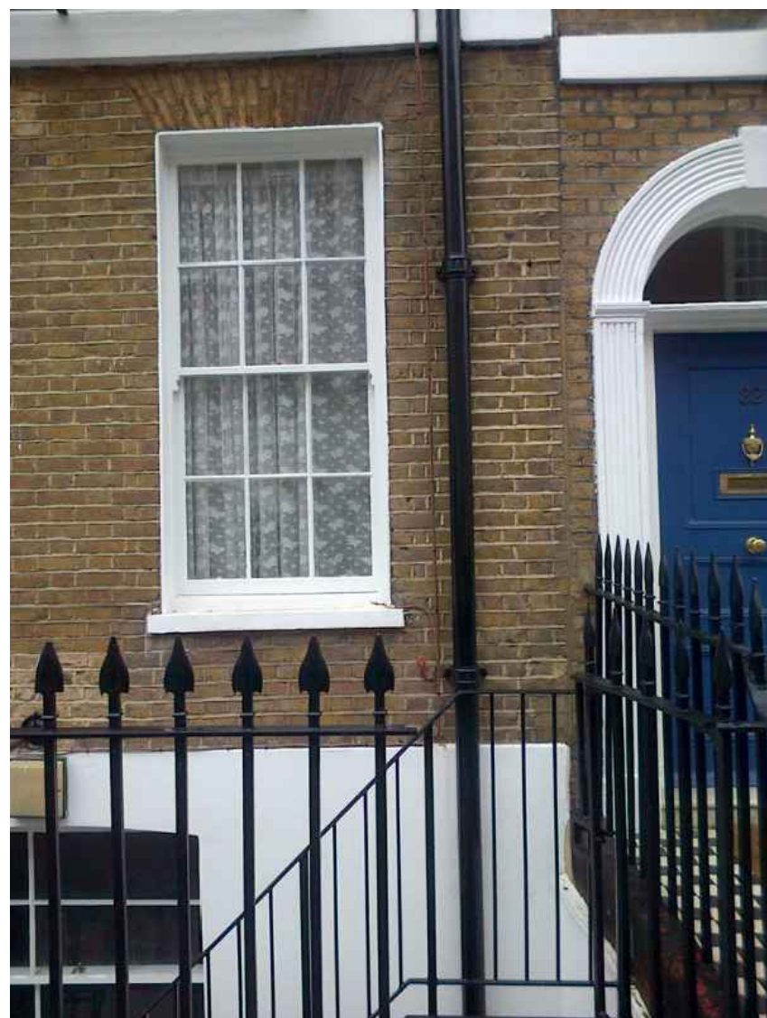
EDGE OF NO.31 POST COMPLETION
