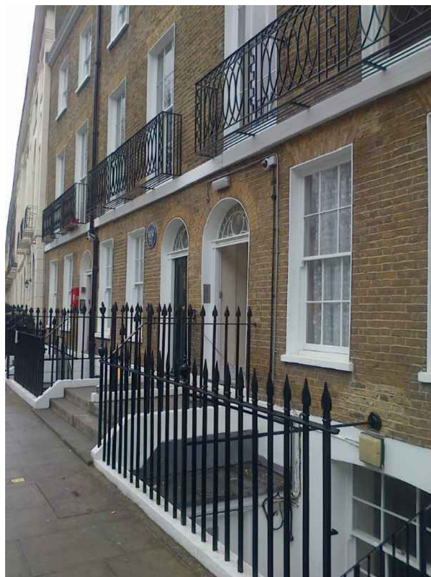
ENTRANCES TO NO. 30 & 31 POST COMPLETION
