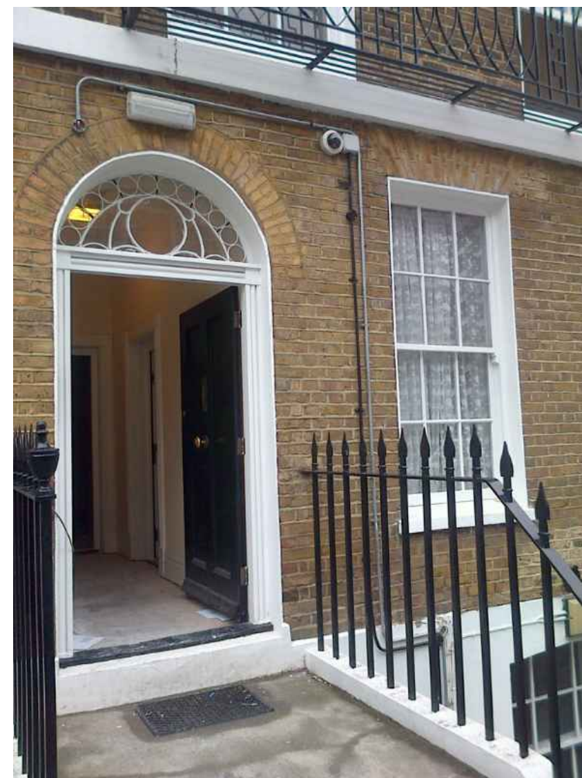
ENTRANCES TO NO. 31 POST COMPLETION
