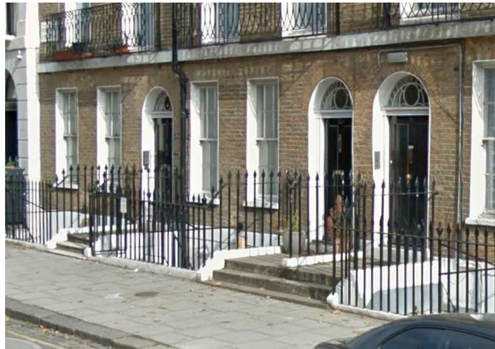
- ENTRANCES TO NO 29, 30 & 31 PRE COMPLETION
