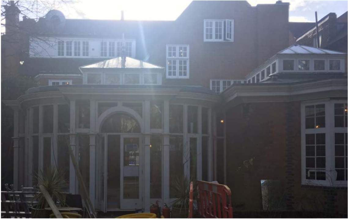
Conservatory with skylights at rear of house.
