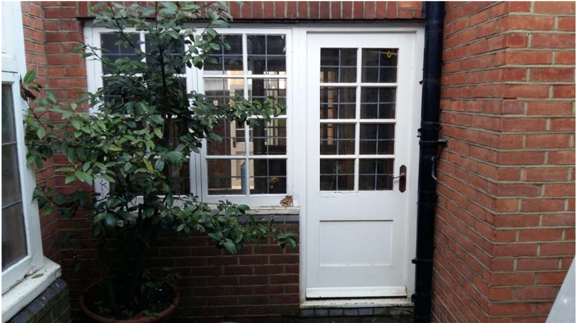
Internal courtyard- east elevation.
