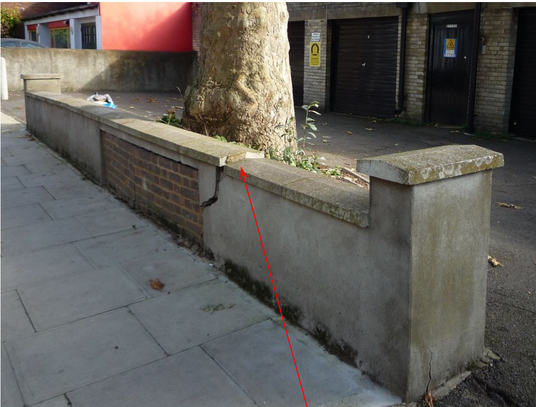
1) Wall in October 2014
