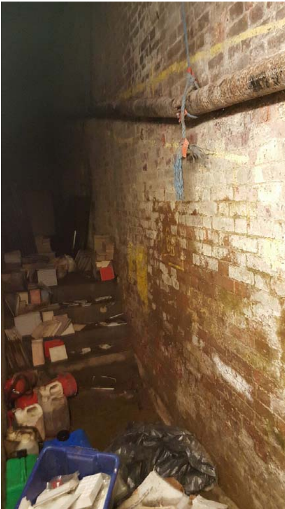
View looking towards Calthorpe Street from within subterranean space
