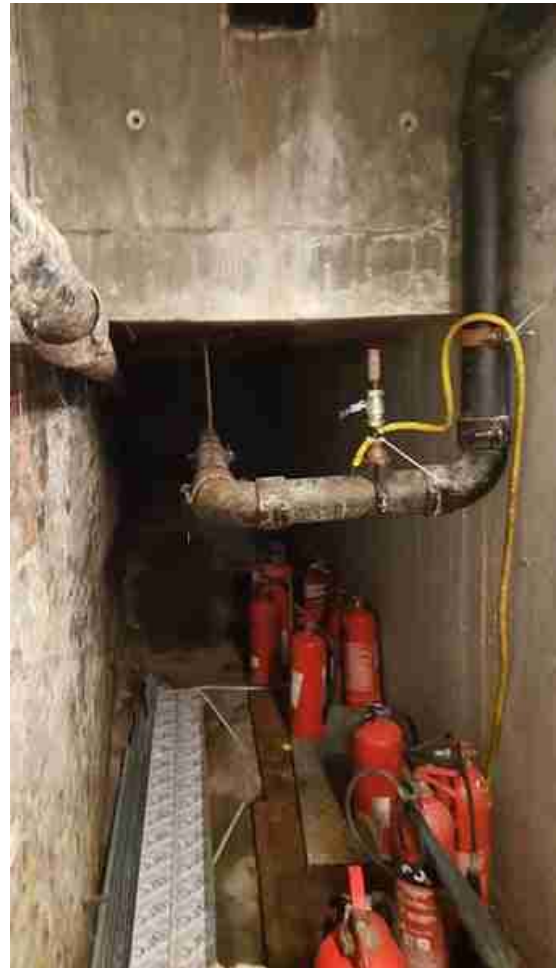
Photo 2: View of rear of the subterranean space between Holiday Inn and 51 Calthorpe Street.
