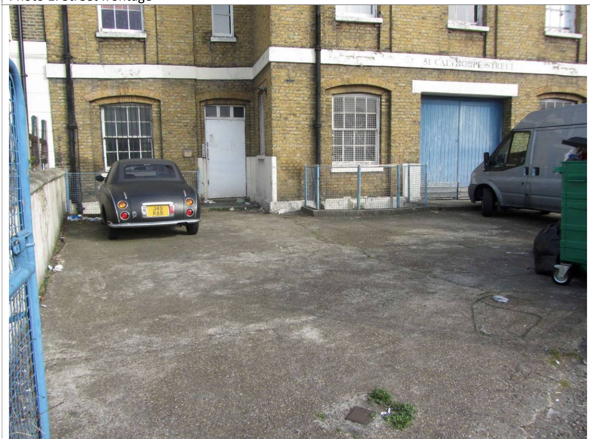
Photo 2: Front hardstanding courtyard & boundary with No.49
