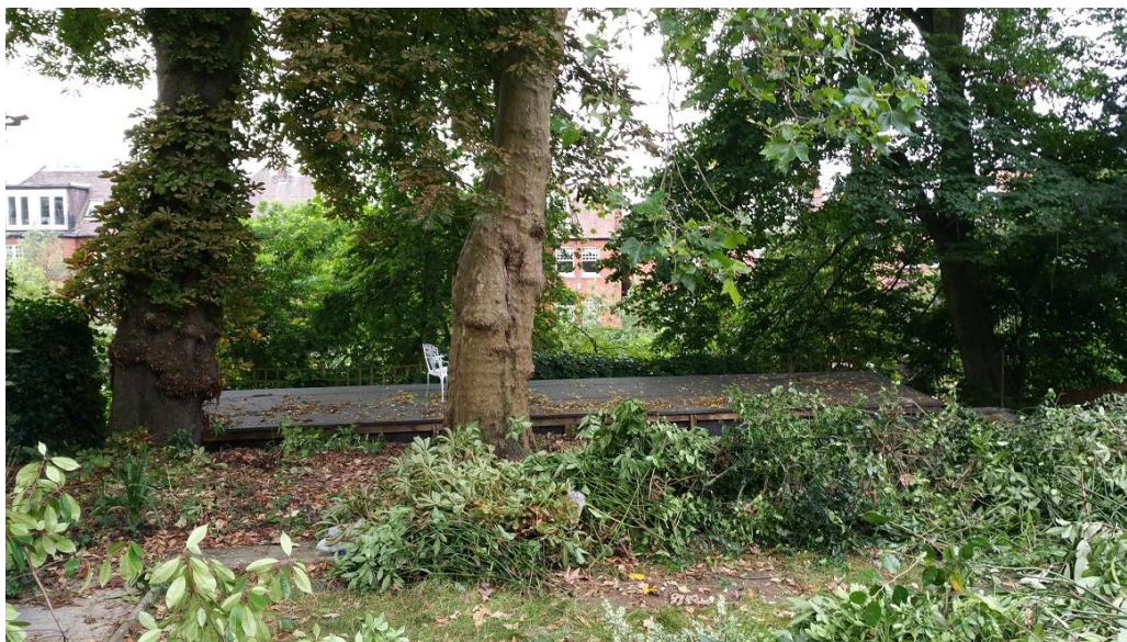
Photo 1 – Garden terrace area prior to installation of timber deck and glass balustrade.
