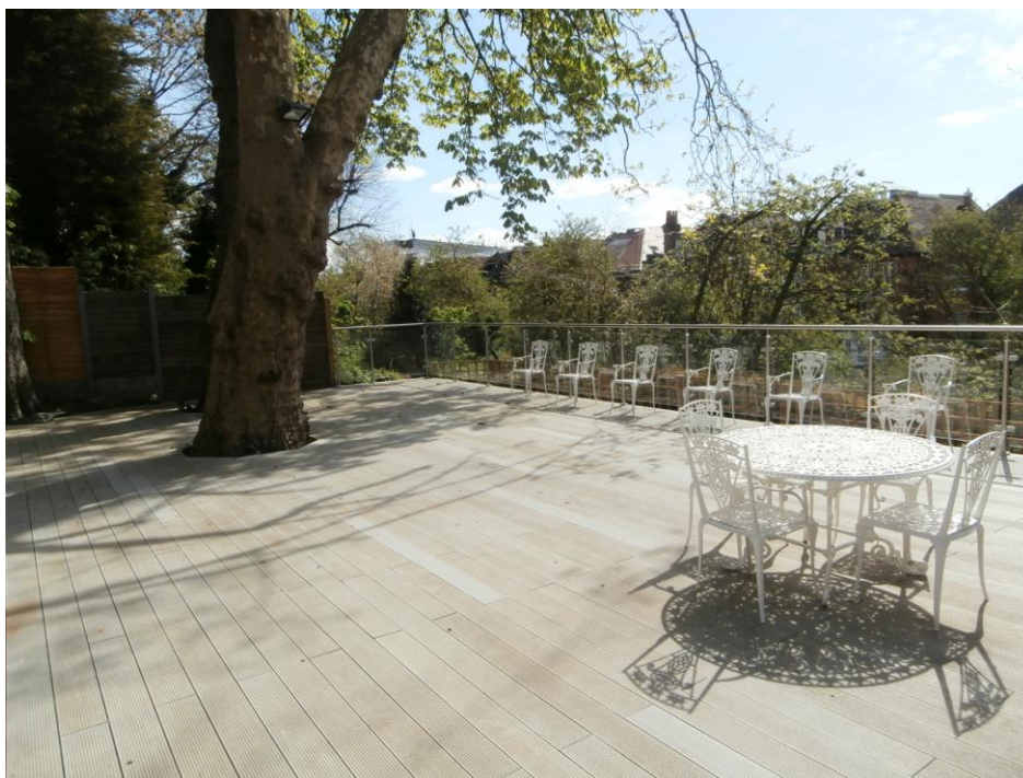
Photo 2 – Timber deck & glass balustrade.
