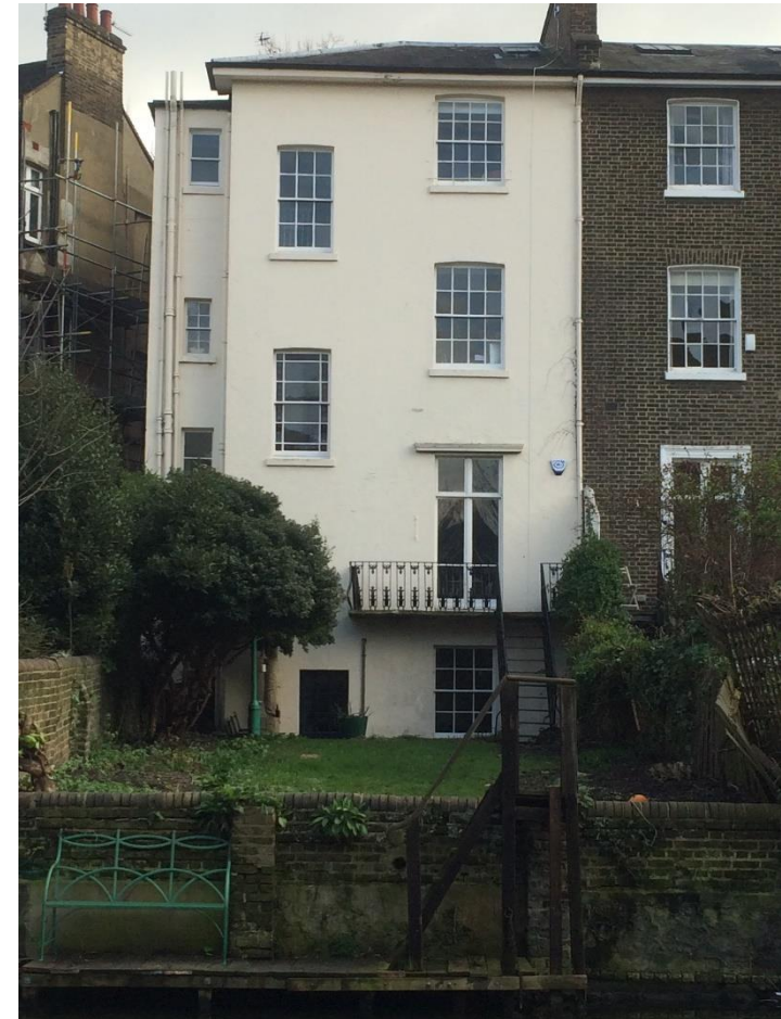
Left: View down front lightwell to level of BH1
