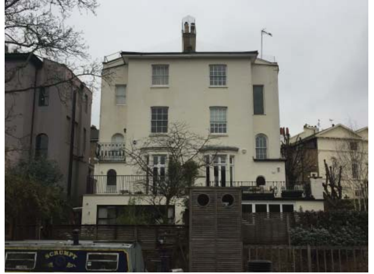
Rear elevation of Nos 14 & 15
