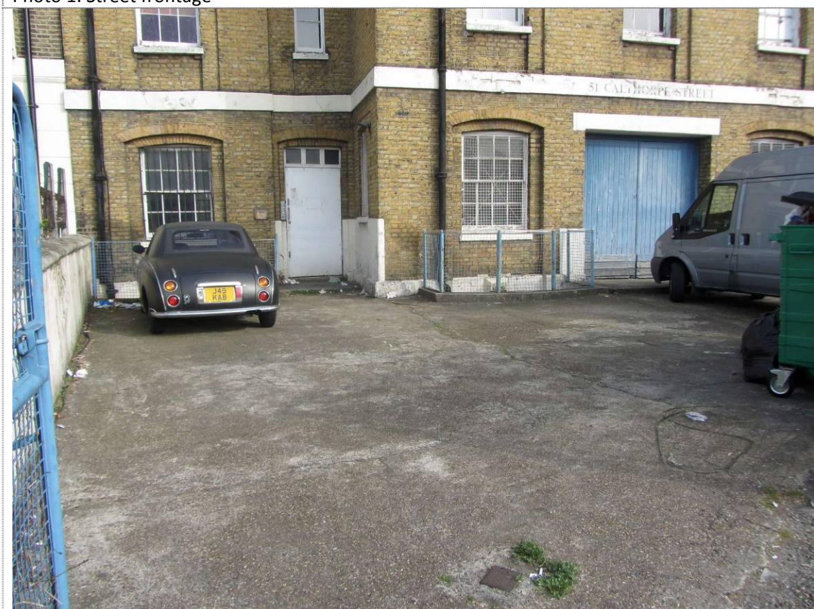
Photo 2: Front hardstanding courtyard & boundary with No.49
