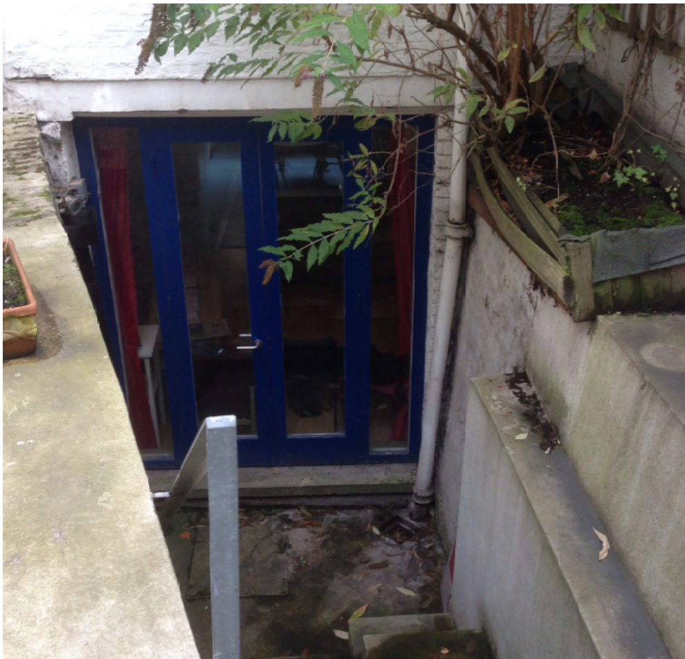
Existing Rear Elevation Lower Ground Floor Window
