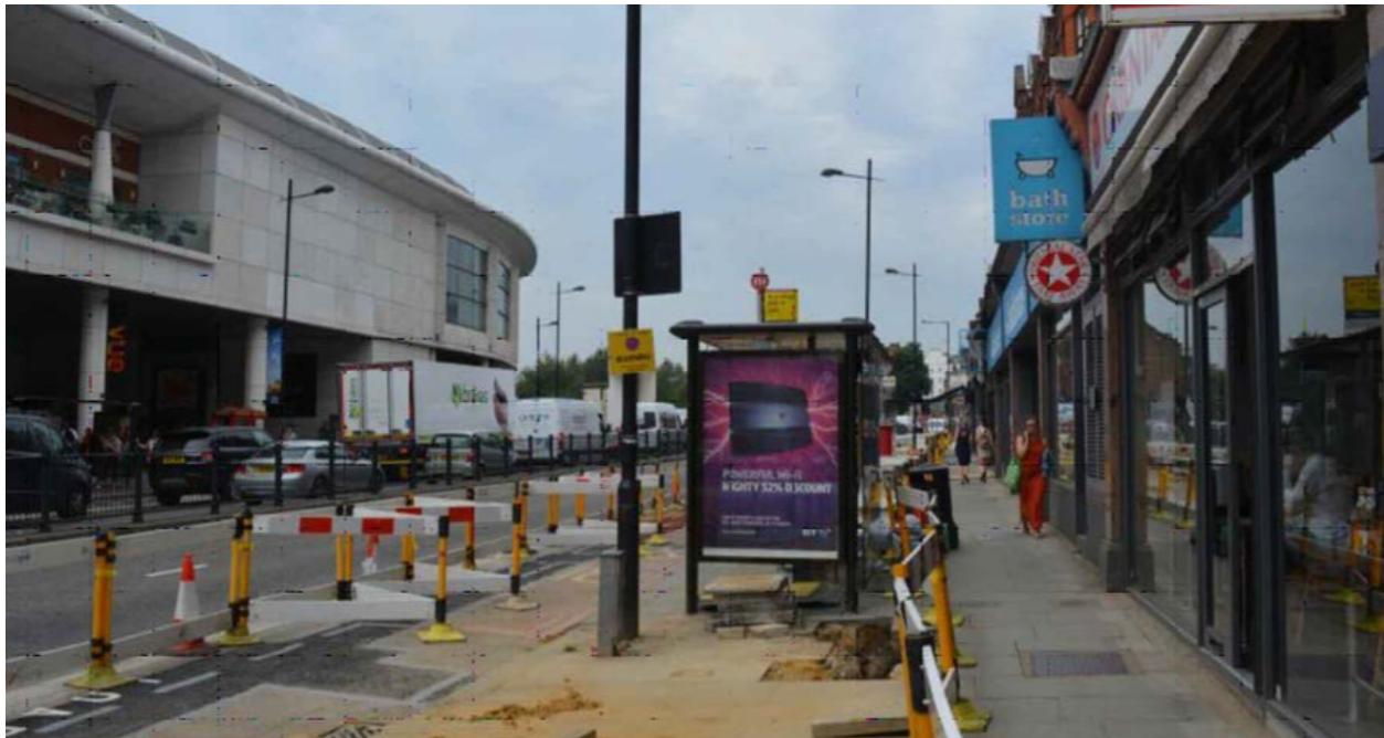
Figure 2 – facing north-west towards Finchley Road and Frognal station
