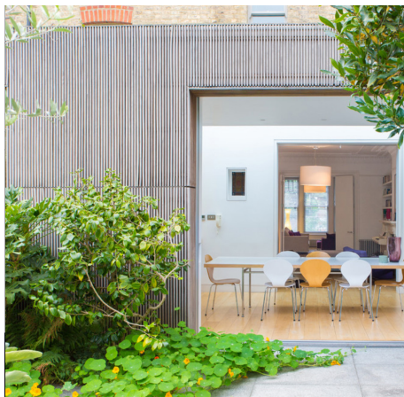
Example of silvered larch cladding
