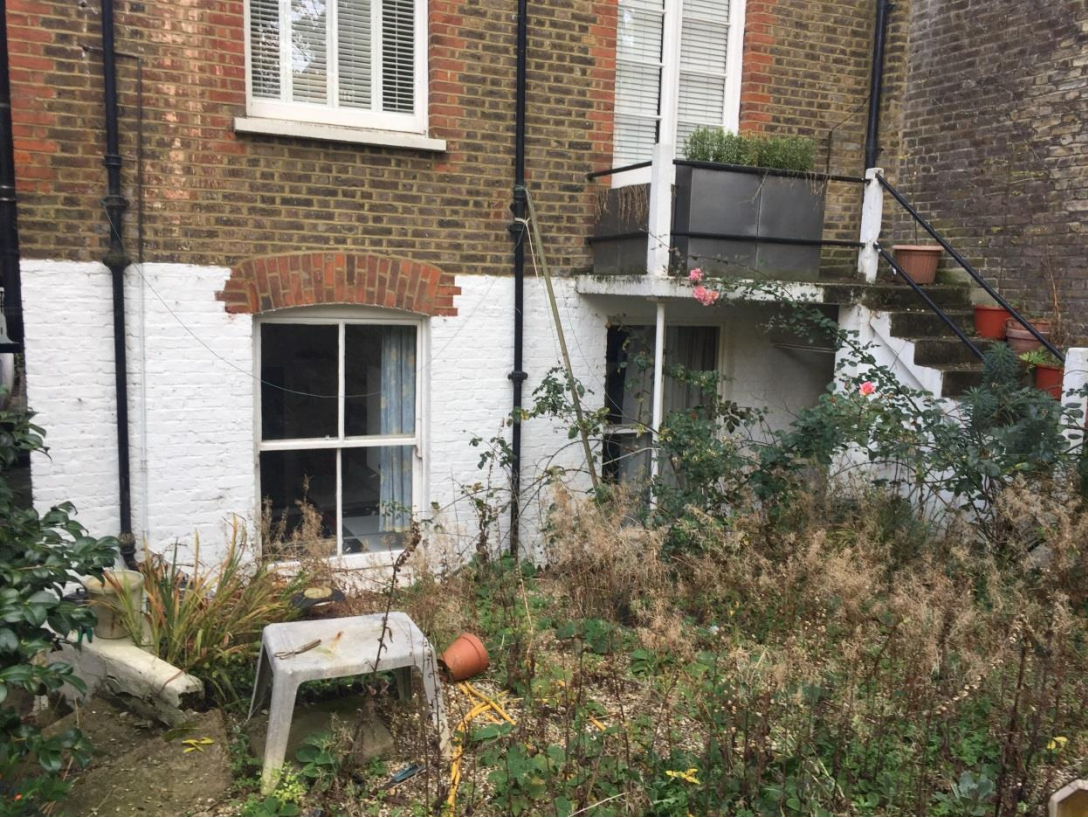
Photo 1: Rear of 134 Fellows with existing roof terrace
