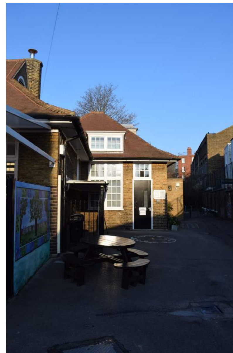
View towards existing KS1 building
