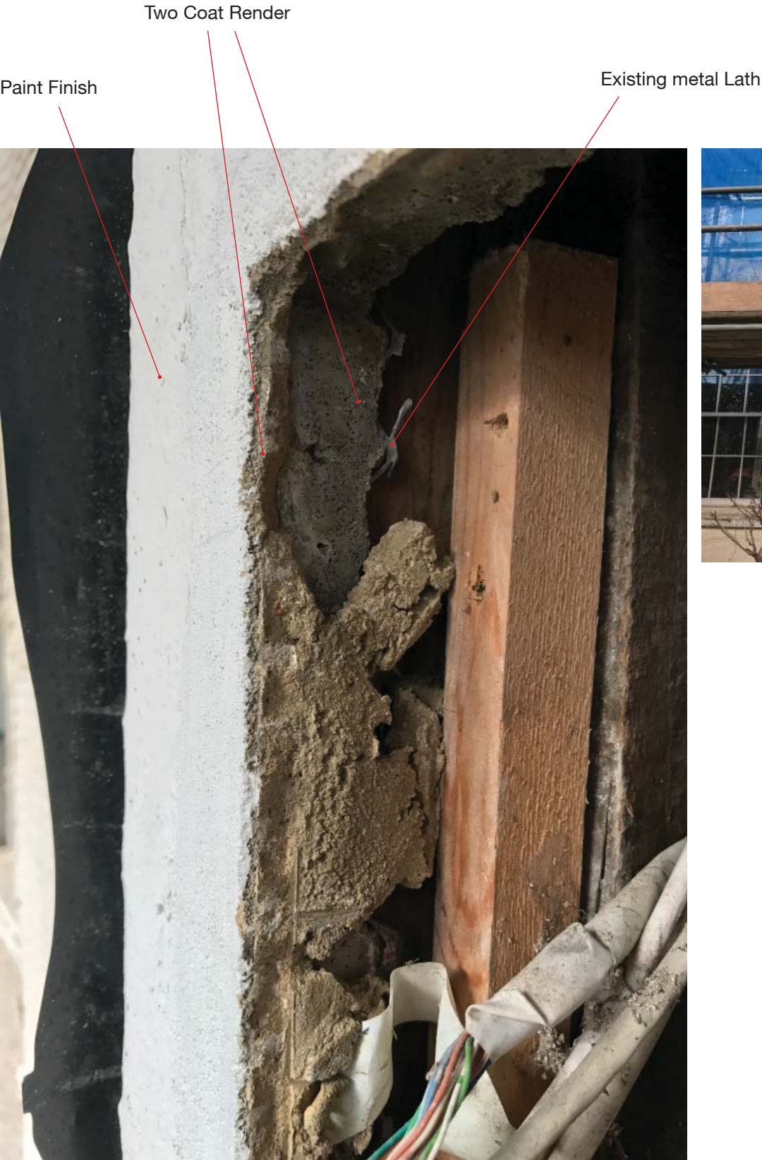
Existing Cut Out At Entry Phone
