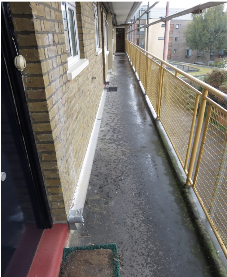
Access deck on the north block showing raised threshold at the entrance door
