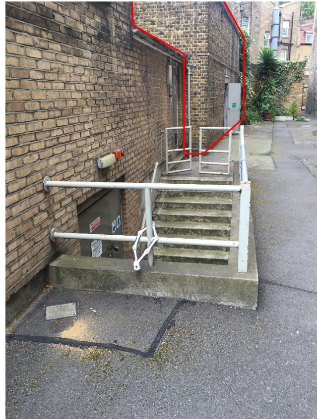
Site Photo 1 Derby Lodge (South Boundary) Photo facing East
