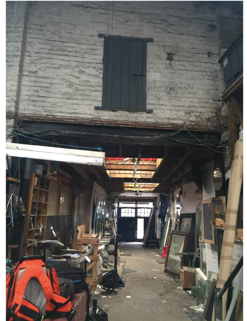
02 Internal photograph showing the restrictive and single entrance to site
