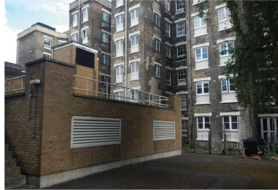
04 View of the boiler house towards Derby Lodge
