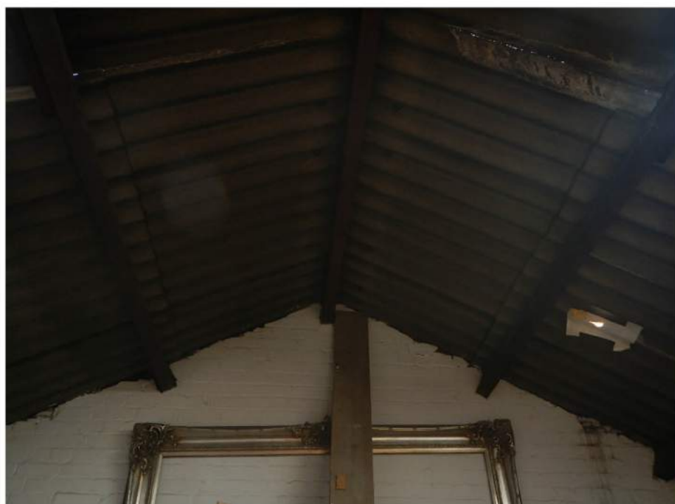
01 View towards the pitched, non-original roof of the warehouse
