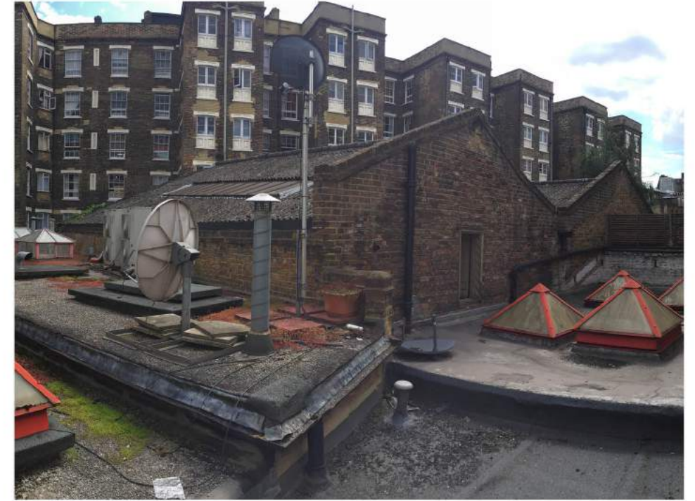
06 External photograph looking towards the existing roof
