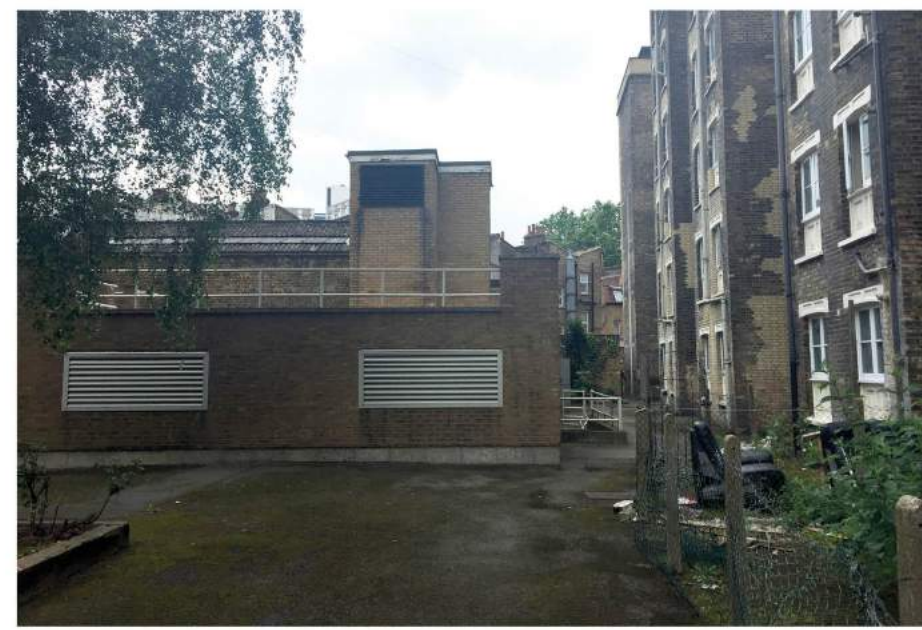
05 View towards the site from Derby Lodge
