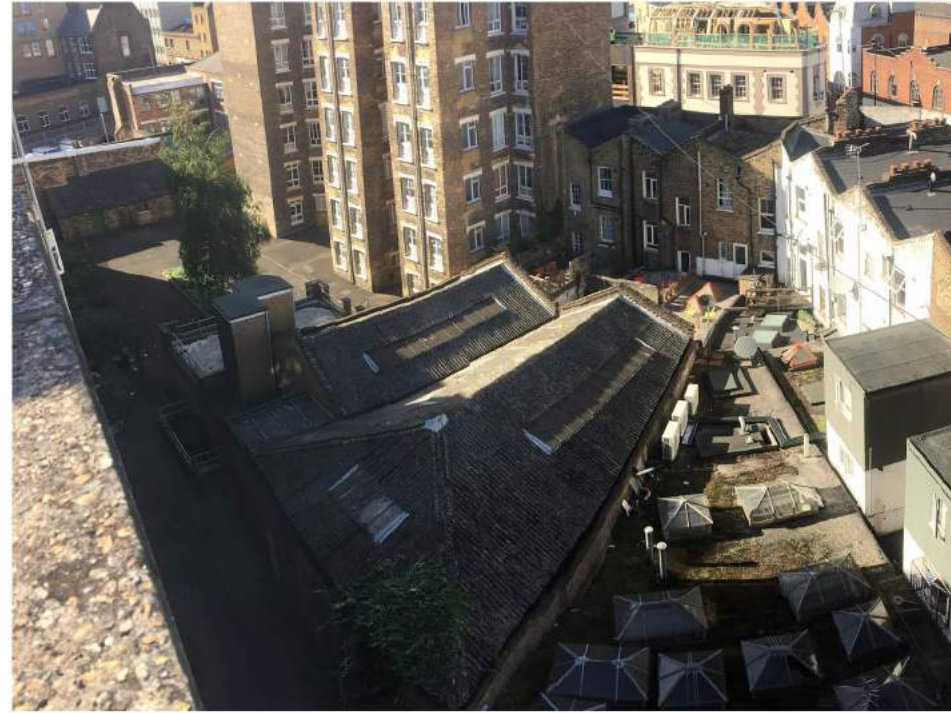
05 External Photograph showing the existing roof
