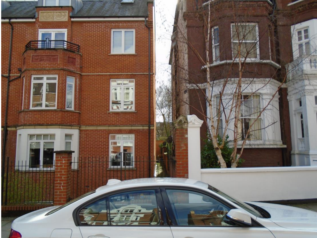
Figure 3. The proposed first floor extension would be glimpsed through the gap between Flats 1-9 Highfield Mews and 75 Compayne Gardens.
