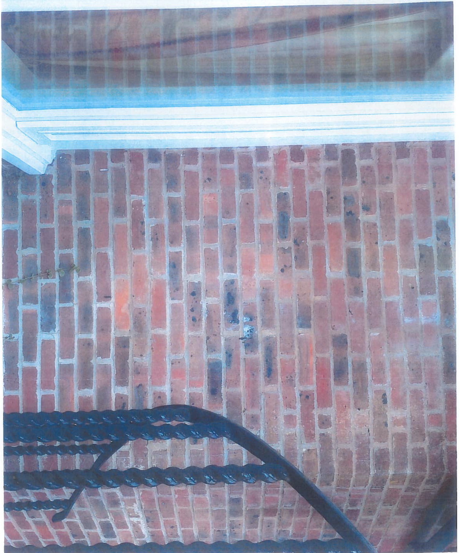
BRICKWORK REAR GARDEN NO. 15 WELL ROAD
