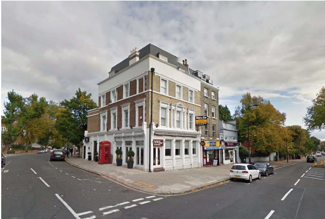
JW4 View of group from NW, existing front of 150 obscures most of No. 148.
