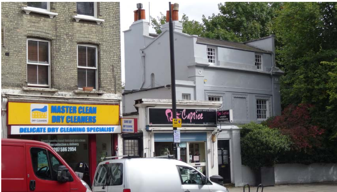
JW3 View from NW, impact of existing front of 150 on setting of 148 villa.
