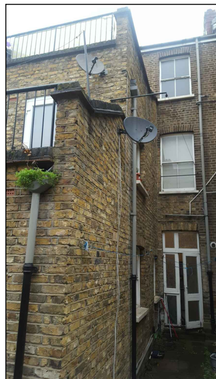
REAR ELEVATION PHOTO
