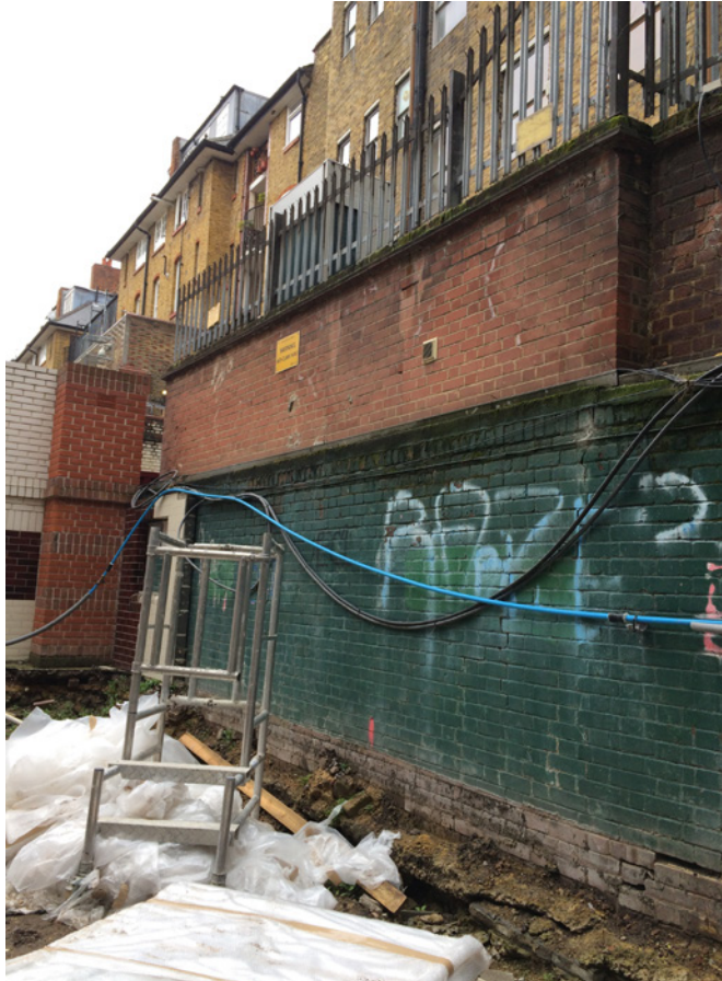
The parapet walls between ownerships vary in height and are capped with galvanised metal security fencing.
