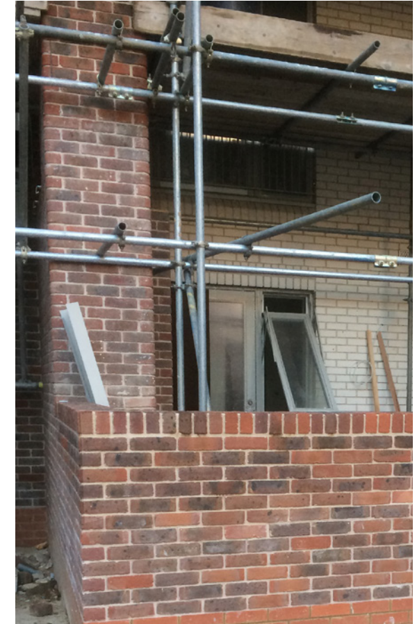
Brick garden wall matches brickwork to block 2:First Quality Multi by Freshfield Lane.
