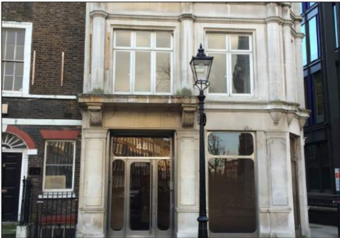
Photo 2: Office entrance on Bedford Row
