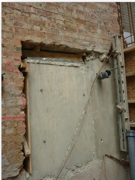
Underpinning To A Party Wall
