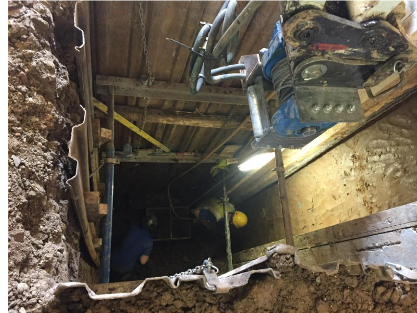
Shored Excavation for an underpin
