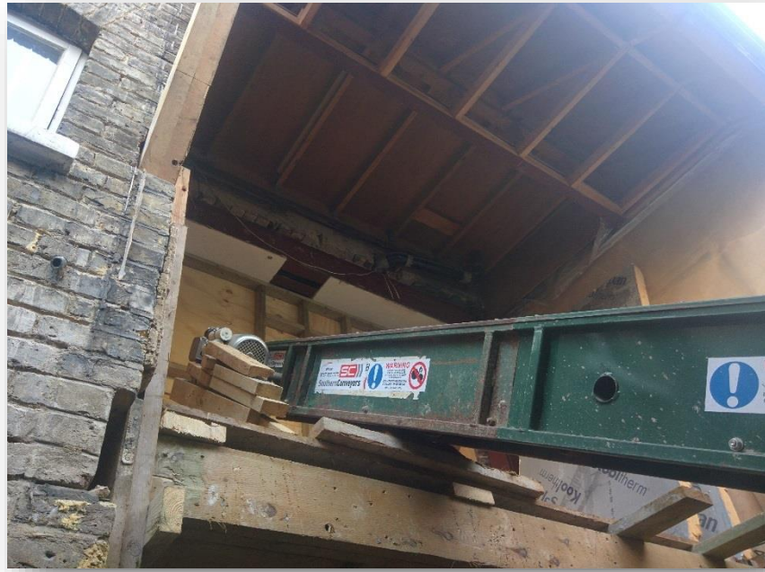
Conveyor to Remove Excavation Arisings
