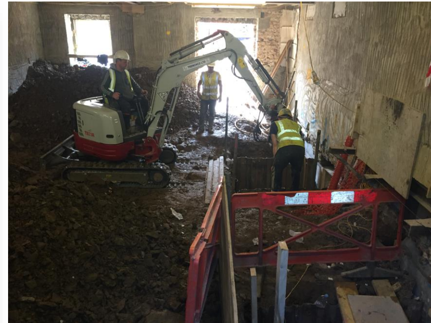
Typical arrangement o underpinning works
