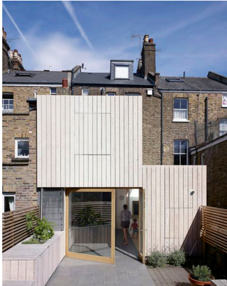
Example of timber cladding
