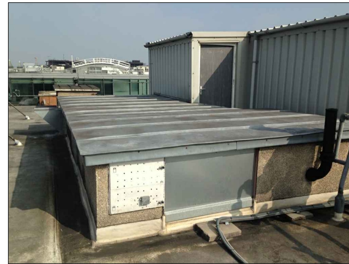
Existing AHU Enclosure
