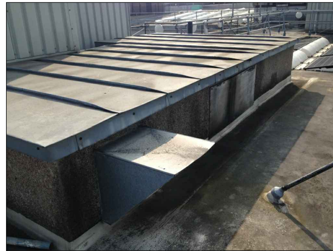
Existing AHU Enclosure
