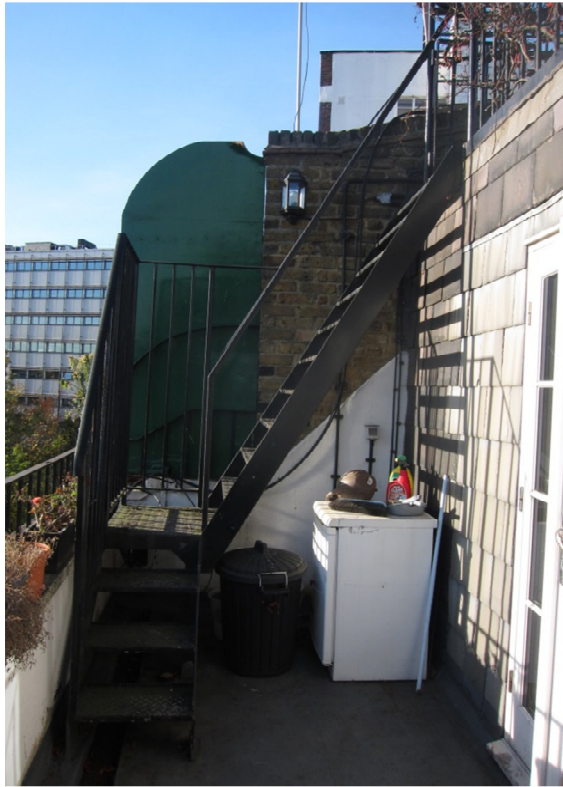
The metal stair to access the roof terrace
