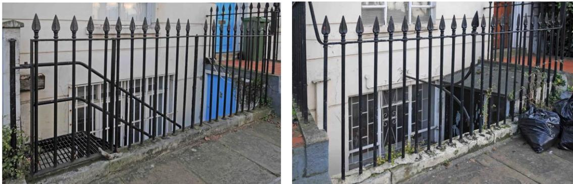
Fig. 3 [Left] Railings, steps, external security grille, mullioned window & plain door to No.124
