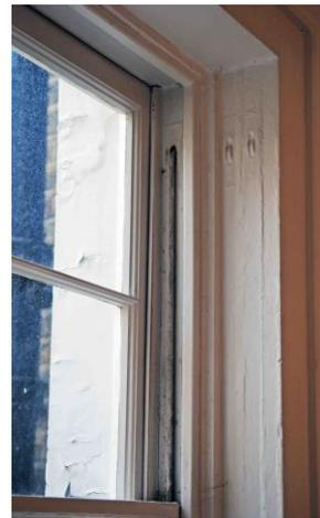
Fig.16 Former vertical shutters to rear ground floor window
