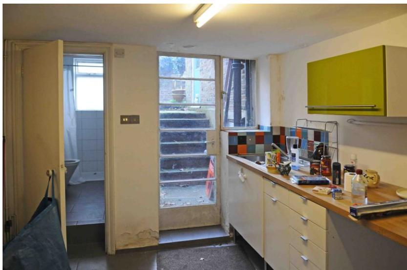
Fig. 12 Basement rear room and toilet/shower extension left. Some penetrating dampness is evident at the base of the rear wall (centre)
