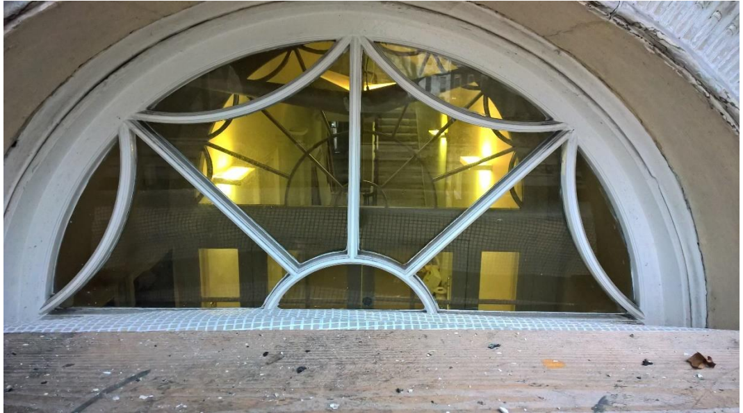
Existing recent timber and plate glass fanlight at No. 48
