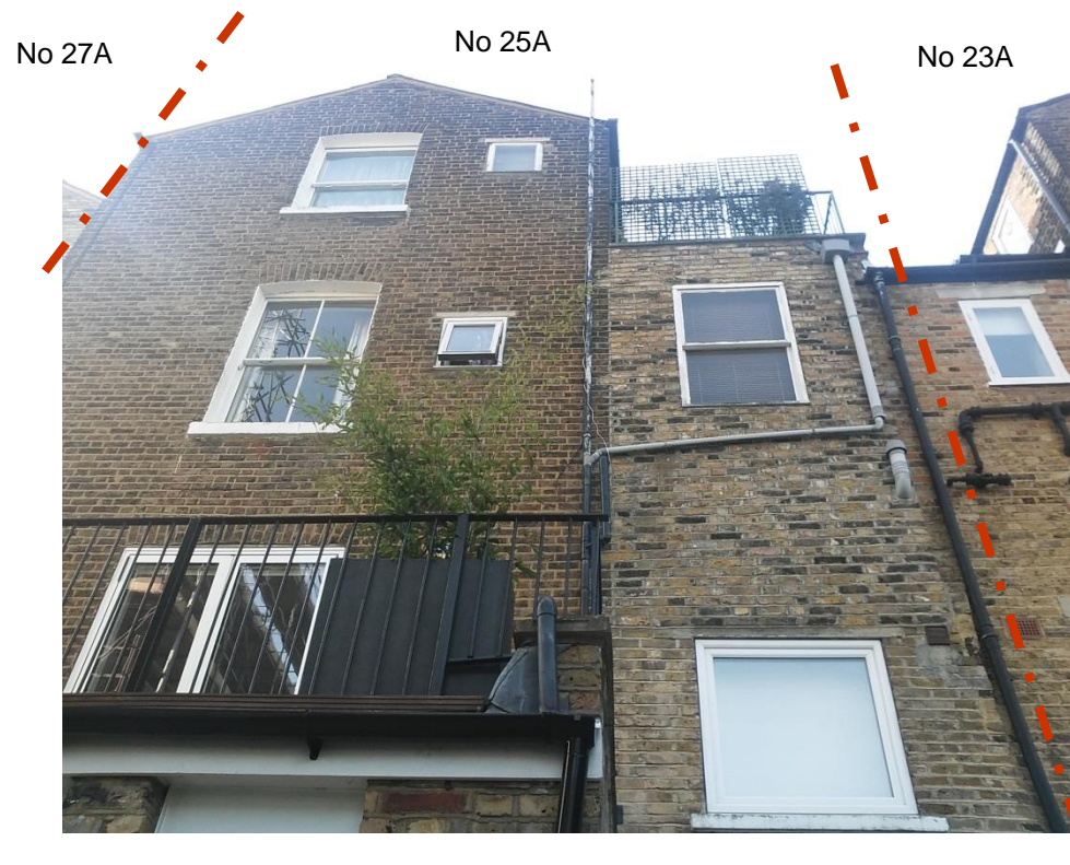
No 25A King Henry's Road Existing Rear Elevation
